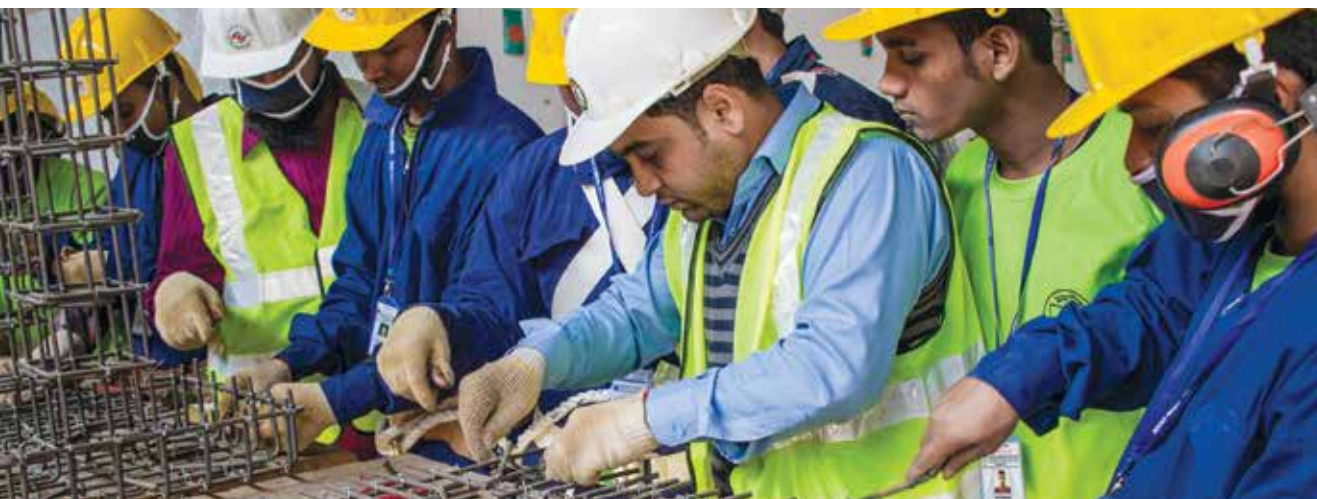
Instructor demonstrating rod binding works for reinforcement of base/footing and column to the participants
